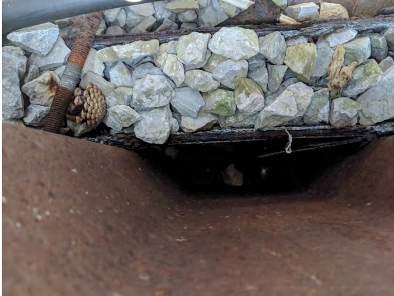
Photo 7 – Segment 2 - Fill Material Behind Wall
