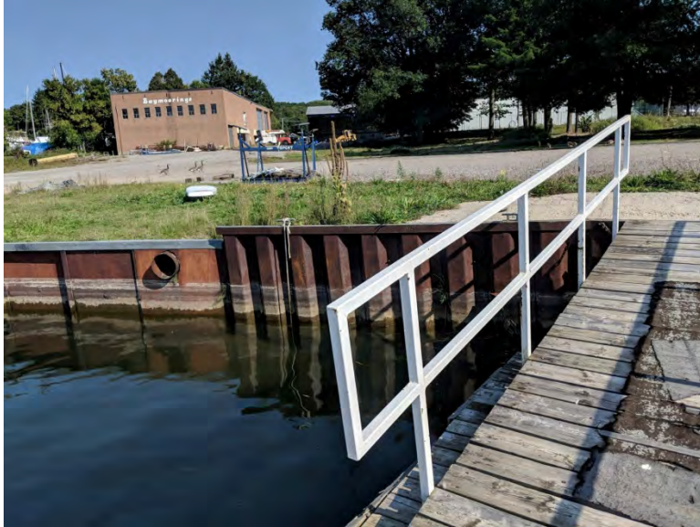
Photo 18 – Segment 7 – Transition to Steel Plate Wall
