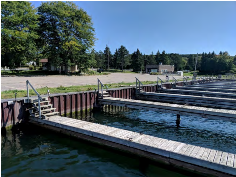
Photo 6 – Segment 2 – Dock Extending from Sheet Pile Wall
