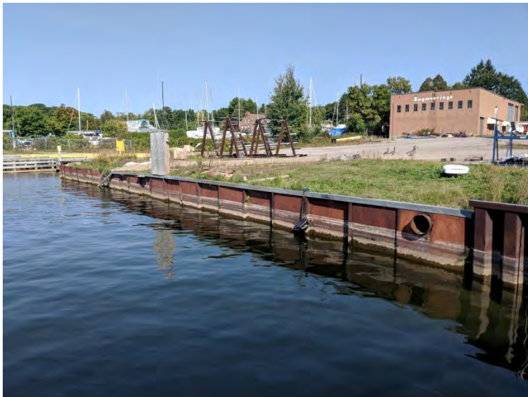
Photo 19 – Segment 7 – Steel Plate Wall
