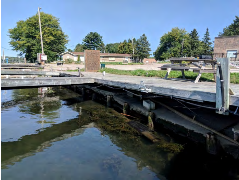
Photo 3 – Segment 1 – Concrete Cap on Timber
