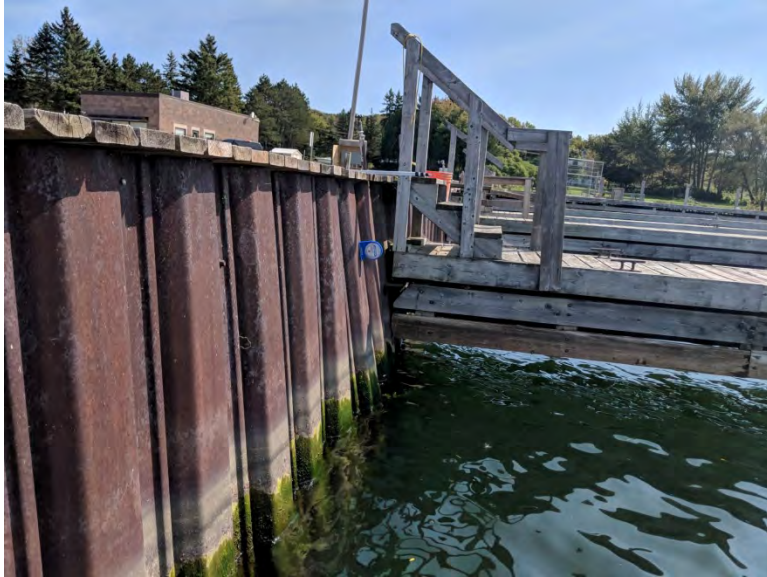
Photo 5 – Segment 2 – Sheet pile wall
