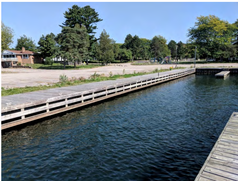
Photo 15 – Segment 6 – Timber Faced Timber Deck In Front of Wall
