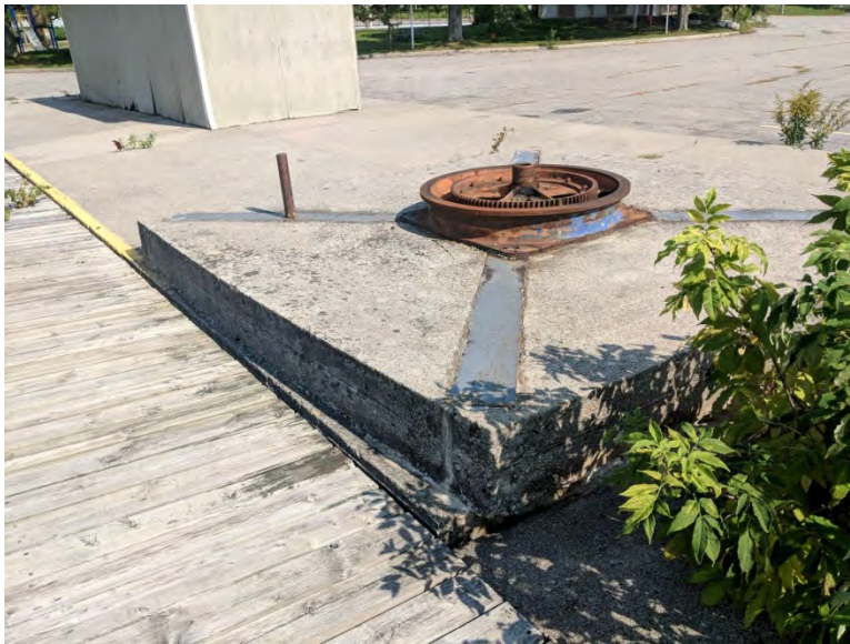
Photo 11 – Segment 3 – Concrete Pad
