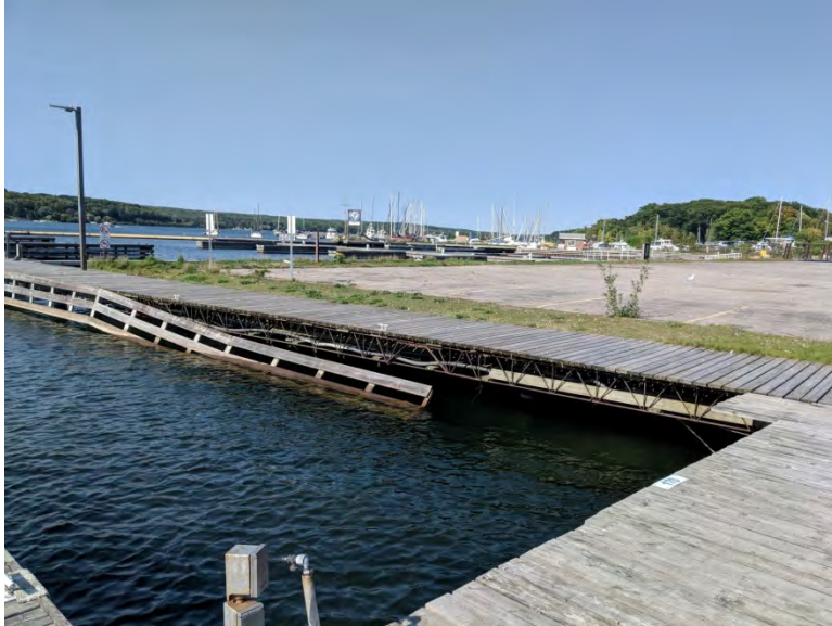
Photo 16 – Segment 6 – Timber Deck In Front of Wall
