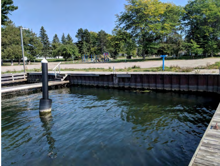
Photo 14 – Segment 5 – Steel Sheet Pile Wall
