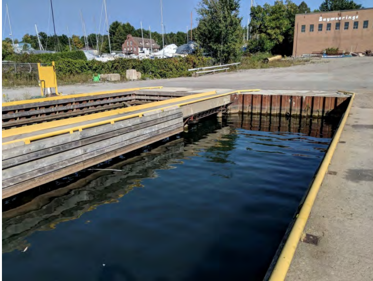
Photo 20 – Boat Slip Wall
