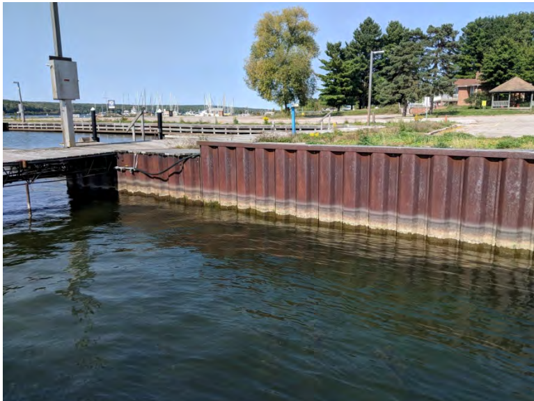
Photo 13 – Segment 4 – Lower End of Wall
