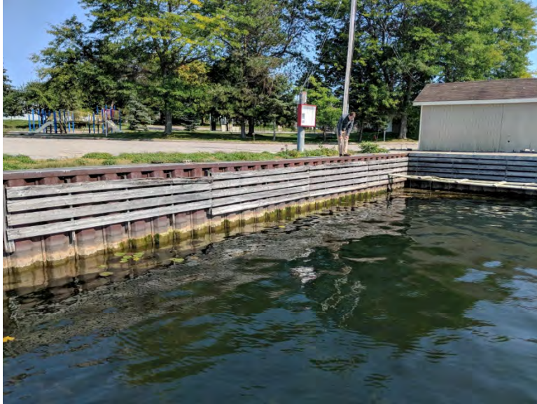
Photo 12 – Segment 4 – Steel Sheet Pile Wall
