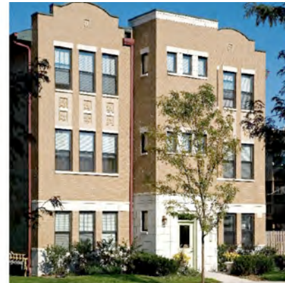
Example of a building with facade articulation that makes it visually more appealing, while still being relatively simple in design and ornamentation. Source: CNU
