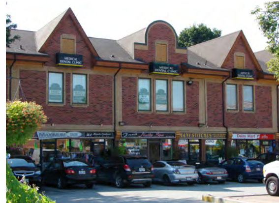
This building uses varied roof lines, pilasters, and window pattern to break up the lengthy facade.
