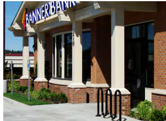
Bike parking located adjacent to a main entrance and visible from inside the building. The bike rack is also located to provide clear pedestrian movement along the walkway.
